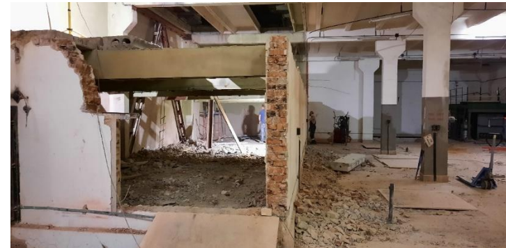
Initial stage of building
